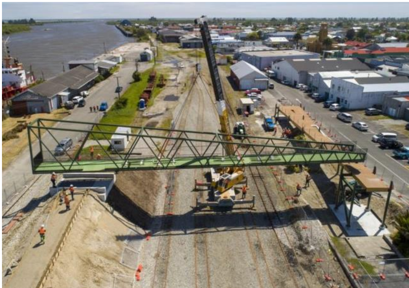
(a) Site view of the Toki Poutangata bridge.
