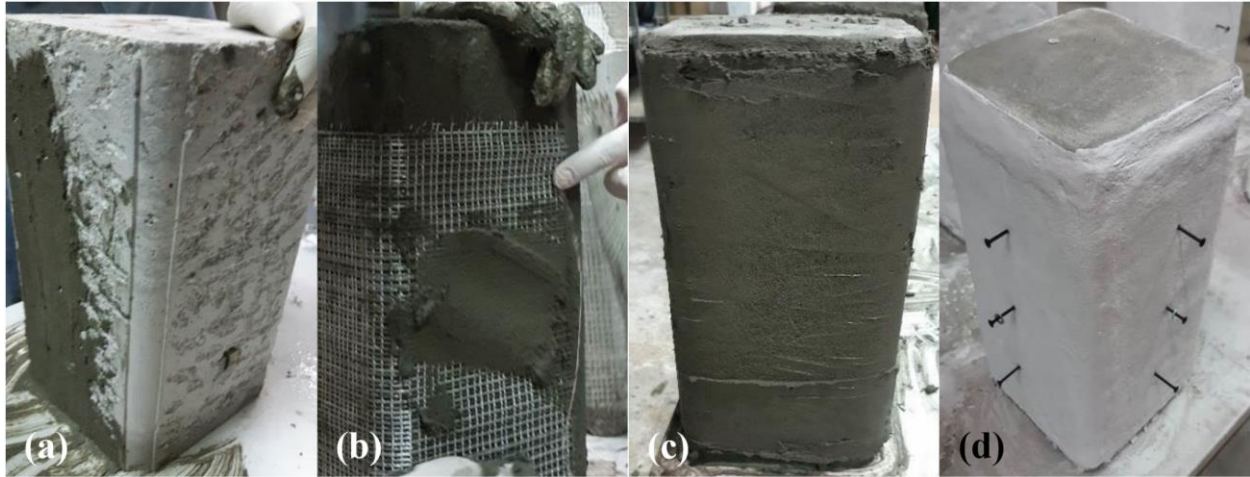
Figure 3. Application of one layer of SRG jacket. a) Application of the first layer of grout; b) Application of the steel textile; c) Application of the second layer of grout; d) View of the retrofitted specimen before testing.
