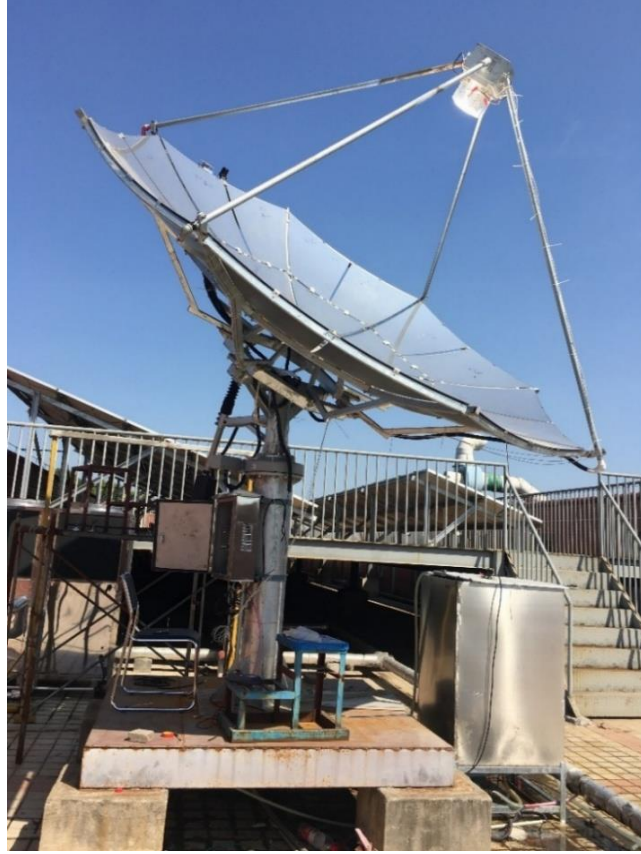
Figure 5: Dish-type concentrator photovoltaic system
