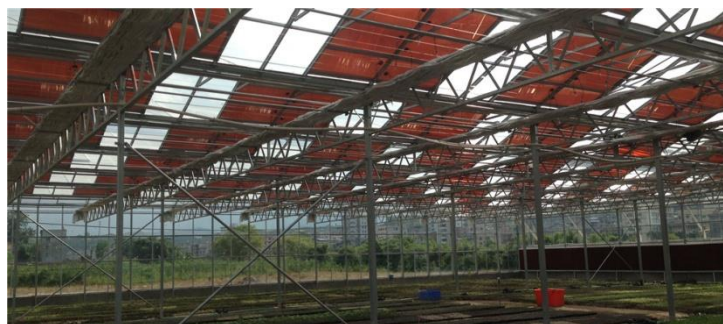
Figure 2: A photovoltaic agricultural project leveraging thin film solar cells
