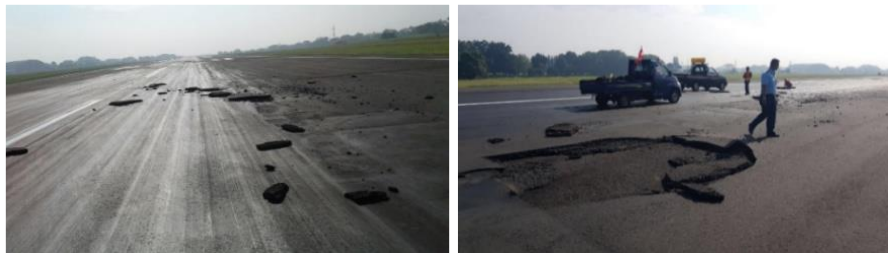
Figure 5. Failure in new asphalt overlay at runway (Courtesy of Indonesia Airport Authority).
