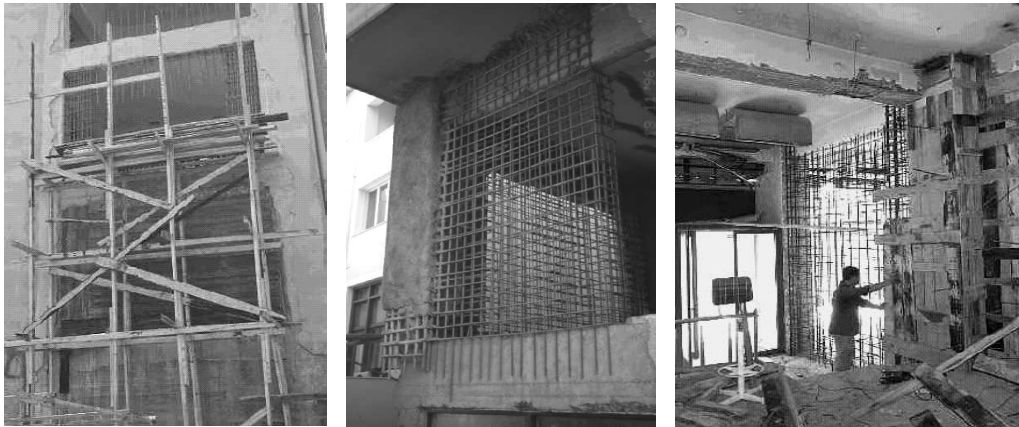
Fig. 5 Cast-in-place infill walls
