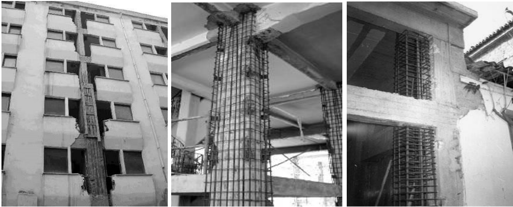
Fig. 4 Reinforced concrete jacketing technique
