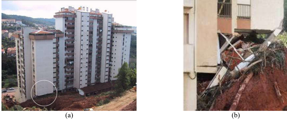
Figure 1 –Severely damaged RC residential building after a land slide: (a) rear façade; (b) collapse of the outer columns of the rear body of building.
