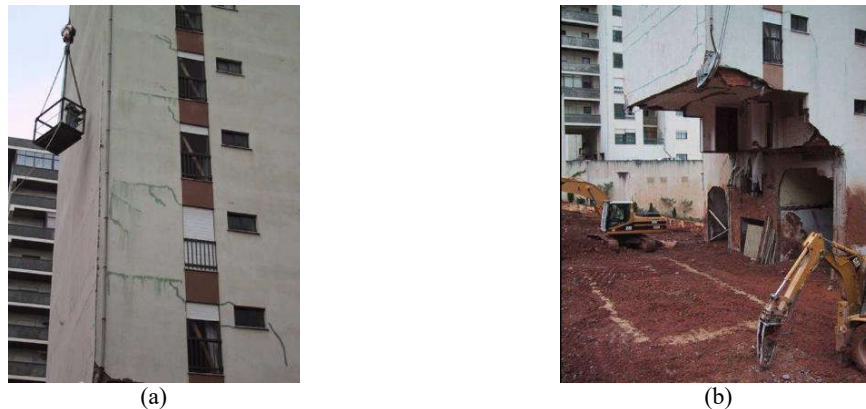
Figure 2 –Details of the accident: (a) cracks along the façade masonry infill walls; (b) removal of debris from the accident site.
