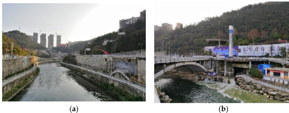
Figure 6. (a) Flood wall on urban reaches; (b) the outlet of the Guan Cheng River Flood Tunnel. Photographed by the authors.
