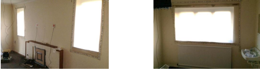
Figure 3: Polyethylene film applied on windows to increase the air tightness of the fabric
