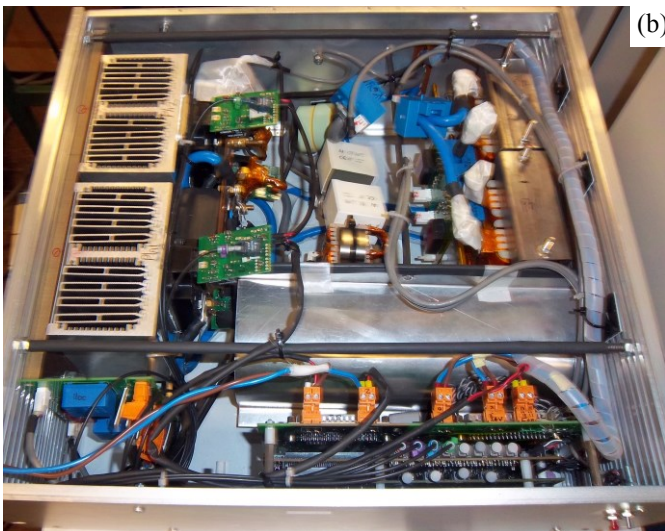
Fig. 14. a) Schematic of the battery energy storage system as connected to a 15kW power supply for testing ; b) Actual implementation of the converter system in a 19" rack enclosure (675x600x200mm) including the EMI filter, cooling, sensors and control boards
