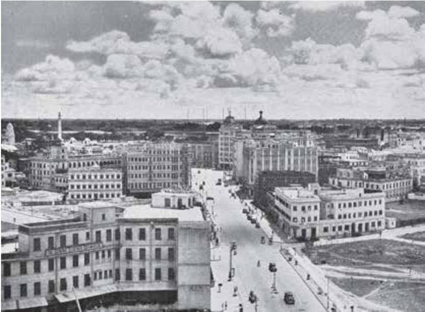
Figure 5.2 Contrasting urban forms in colonial India.
