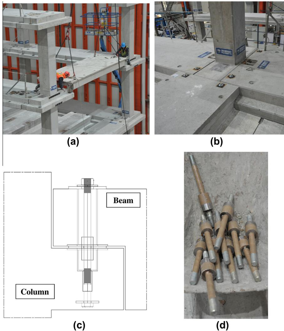
**Fig. 6.** (a) Seating of a secondary beam on the column capital. (b) A central beam–column joint. (c) Detail of a pinned beam–column joint connection. (d) Special dowels with increased diameter at the critical section.
